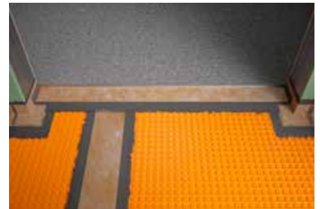
Schlüter-KERDI-CID with sloped covering (slope not to exceed 6%)
