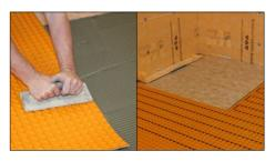
① If Schlüter-DITRA 25 uncoupling membrane, or Schlüter-DITRA-HEAT-E /-DUO underfloor heating is being used apply a bed of adhesive to the floor substrate and adhere the uncoupling membrane.
