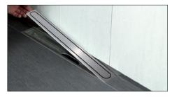
18 Remove the spacer strip and height-adjustment aid after curing. Then insert the grate.
