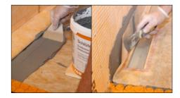
Adhere the Schlüter-KERDI collar, using the sealing adhesive Schlüter-KERDI-COLL-L (see Product Data Sheet 8.4), to the adjoining waterproofing assembly with a 3 x 3 mm or 4 x 4 mm notched trowel and comb provided. Completely embed the KERDI collar in this assembly, observing the curing times of all materials.
