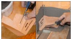
① Cut the supplied Schlüter-KERDI-KERECK inside corner to size and attach it with KERDI-COLL-L.
