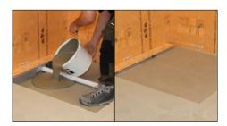
4 Taking into account the height of the Schlüter-KERDI-SHOWER preformed shower board and the height of a bed of tile adhesive, screed a flat area of the same size as the shower board. This is likely to just cover the drain outlet.
