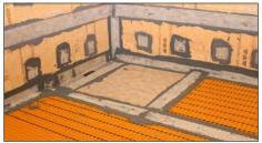
Use KERDI-COLL-L to create tightly sealed wall connections with KERDI-KEBA sealing band.
