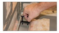
Use the supplied height-adjustment aid to adjust the frame to the thickness of the tile covering.
