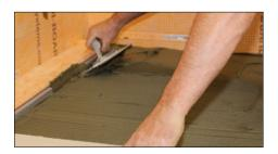
6 Apply a bed of tile adhesive to the surface of the dry screed, ensuring the front edge of the drainage channel has adhesive underneath it.
