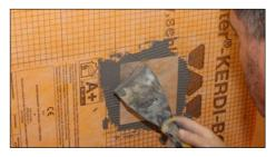
(2) If Schlüter-KERDI-BOARD is used on the wall, use KERDI-COLL-L with a piece of Schlüter-KERDI-KEBA sealing band to waterproof the penetrations.
