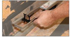
(5) Insert the frame with the spacer strip. If the 30mm high frame is being used (only suitable for use with a central outlet position) carefully adjust the grate support feet around the trap so the trap can be removed for cleaning.
