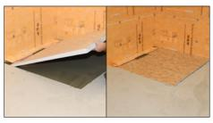
3 Carefully place the KERDI-SHOWER preformed shower board on top of the adhesive bed, sliding the tray under the flange of the drainage channel. Care should be taken to ensure the channel is not lifted.
