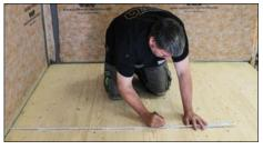
2 Mark on the floor the outline of the Schlüter preformed shower tray to be fitted. This may be influenced by the position of the floor joists and by your use of an uncoupling membrane or underfloor heating in the surrounding floor area. For example, with an 18mm thick timber floor, a Schlüter preformed shower tray cut to 1000mm long creates a flush level access shower area when Schlüter-DITRA-HEAT-DUO is installed in the surrounding area.
