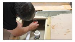
Oconnect the drain outlet to the building drainage system ensuring an appropriate fall on the waste pipe. Check for leaks. Using a spirit level, check the drain is still level along its length and across its width, adjusting if necessary.
