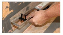
29 Insert the frame and spacer strip. If the 30mm high frame is being used (only suitable for use with a central outlet position) adjust the grate support around the trap to allow for cleaning.
