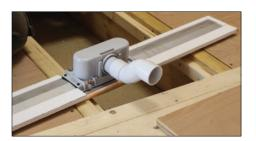
(B) Remove the drain and using solvent weld adhesive glue bends, as appropriate, to the outlet of the drain. One Floplast WS19 135° (45°) bend and one Floplast WS77 135° (45°) conversion bend usually works well.
