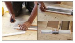
Cut the white polystyrene channel supports to size, ensuring they will fit tightly up to either side of the drain body/sump. Cut the adhesive tape to size and adhere to the underside of the drain. Carefully attach the polystyrene channel supports to the adhesive tape, ensuring they are firmly attached to the underside of the drain.
