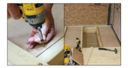
Screw fix the sub-floor to the battens, ensuring it is level. At this stage do not fix battens or the sub-floor to the area where the drain body/sump will be installed.
