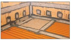
28 Use KERDI-COLL-L to create tightly sealed wall connections with KERDI-KEBA sealing band.
