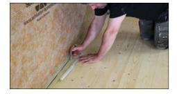
1 Identify and mark on the floor the position of the floor joists. The position of the screws or nails in the floor should provide an indication.
