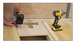
Using screws, secure the longer piece of plywood to the battens described in step 8.
