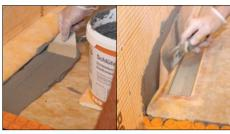
Adhere the Schlüter-KERDI collar, using the sealing adhesive Schlüter-KERDI-COLL-L (see Product Data Sheet 8.4), to the adjoining waterproofing assembly with a 3 x 3 mm or 4 x 4 mm notched trowel and the comb provided. Completely embed the KERDI collar in this assembly, observing the curing times of all materials.
