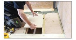
2) Place the remaining part of the sub-floor into position, screw fixing the shorter of the two pieces of plywood cut in step 16 to the battens. The longer piece should be placed on top of the lower piece and on top of the 'ledge' described in step C on page 4, or as part of the G3 Installation Accessory 'KLF43G3TA'. The top piece should then be screwed to the bottom piece.
