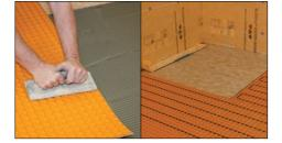
If Schlüter-DITRA uncoupling membrane, or Schlüter-DITRA-HEAT-E /-DUO underfloor heating is being used, apply a bed of adhesive to the floor and adhere the membrane. As per Product Data Sheet 6.1, a 3 x 3 mm or 4 x 4 mm notched trowel should be used to install DITRA. As per Product Data Sheet 6.4, a 6 x 6 mm notched trowel should be used to install DITRA-HEAT-E/-DUO.
