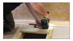
If strengthening the sub-floor as described on page 4 (and not using the pre-built G3 Installation Accessory 'KLF43G3TA') screw fix it into the supporting battens described in step 8, ensuring it finishes flush with the top of the joists. Otherwise proceed directly to step 18.
