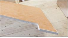
Outline a utility knife and the pre-printed markings on the back, measure and cut out the sloped tray Schlüter-KERDI-SHOWER KSLT13652000S to accommodate the drainage channel. If the drainage channel is fitted away from the wall ensure it still fits within the level end of the tray, and use either 12.5mm thick KERDI-BOARD, or the offcuts from the level end of the tray, to infill the gap between the wall and the tray.
