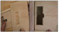
1) Take the shorter piece of plywood from the box containing the G3 Installation Accessory 'KLF43G3TA' and position it over the piece of plywood cut-to-size in step 10. The rectangular openings should be aligned and the shorter piece of plywood cut to size so it fits on top of the longer piece and between the joists.
