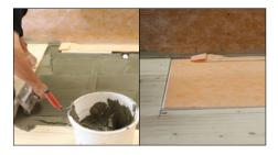
Using an appropriate notched tiling trowel, apply a bed of tile adhesive to the surface of the sub-floor where the shower tray will be installed. Carefully place the preformed shower tray on top of the adhesive bed, sliding the tray under the flange of the drainage channel. Ensure it is solidly bedded, adjusting the trowel size if necessary. Care should be taken to ensure the channel is not lifted.
