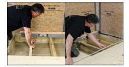
Determine the position of the linear drain in the floor, taking into consideration the position of the floor joists and the size of the shower tray. The drain could be positioned either centrally or offset between the joists, but is usually positioned central to the shower tray width.
