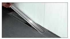
8 Remove the spacer strip and height-adjustment aid after curing. Insert the grate.
