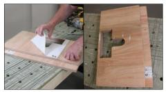
Remove the template used in steps A & B. Place the two pieces of plywood on top of each other ensuring the cut-outs align and glue (using a PVA-based D3 waterproof wood glue such as Gorilla Wood Glue) and screw together. Use screws sized to penetrate the second piece of plywood by at least 10mm. Screws should be no further than 150mm apart across the whole of this piece of strengthened sub-floor. Attach to the battens described in step 8.
