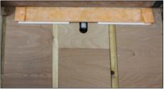
Cut two further pieces of 18mm exterior grade plywood to fit, one on top of the other, in the remaining part of the sub-floor. Check they fit and then remove.
