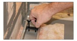
Use the supplied height-adjustment aid to adjust the frame to the thickness of the tile covering.
