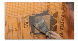
If Schlüter-KERDI-BOARD is used on the wall, use KERDI-COLL-L with a piece of Schlüter-KERDI-KEBA sealing band to waterproof the penetrations.
