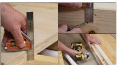
3 Fix supporting battens to the side of the joists in the section of the floor where the drain will be fitted. The top of the battens should be positioned 36mm from the top of the joists. Use screws sized to penetrate the joists by at least 10mm.
