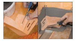
Cut the supplied Schlüter-KERDI-KERECK inside corner to size and attach it with KERDI-COLL-L.
