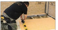
**5** Check the width and length of the Schlüter preformed shower tray to be fitted and using a utility knife, cut to size.
