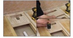
B Position the shorter piece of plywood over the longer piece secured to the battens in step 12, ensuring the routed-out section is face down and the cut-outs align. Glue the two pieces of plywood together (using a PVA-based D3 waterproof wood glue such as Gorilla Wood Glue) and then screw together. Use screws sized to penetrate the second piece of plywood by at least 10mm. Screws should be no further than 150-200mm apart across the whole of this piece of strengthened sub-floor.
