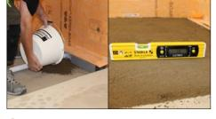
4 Using screed create the slope (between 1 in 35 and 1 in 80) of the shower area, ensuring it is carefully installed up to and against the previously installed and levelled Schlüter-KERDI-LINE-G3 drain.
