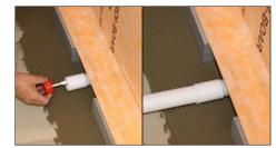
3 Connect the drain outlet to the building drainage system, ensuring an appropriate fall on the waste pipe. Check for leaks.
