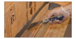
Adhere the Schlüter-KERDI collar, using the sealing adhesive Schlüter-KERDI-COLL-L (see Product Data Sheet 8.4), to the adjoining waterproofing assembly with a 3 x 3 mm or 4 x 4 mm notched trowel and the comb provided. Completely embed the KERDI collar in this assembly, observing the curing times of all materials.
