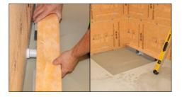
1 Having determined the position of the drain and the outlet, carefully attach the grey polystyrene channel support to the adhesive tape on the underside of the drain, ensuring it is firmly attached.
