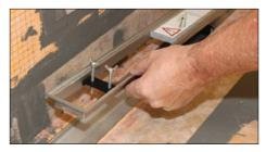
(2) Insert the frame with the spacer strip. If the 30mm high frame is being used (only suitable for use with a central outlet position) carefully adjust the grate support feet around the trap so the trap can be removed for cleaning.
