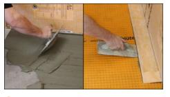
**5** Once the screed is ready to bear weight, solidly embed Schlüter-DITRA, or Schlüter-DITRA-HEAT/-DUO underfloor heating, on the screed area with thin-bed tile adhesive (recommended notched trowel size 3 x 3 mm or 4 x 4 mm). The tile format for installation over DITRA, or DITRA-HEAT/-DUO underfloor heating, must be at least 5 x 5 cm (see Product Data Sheets 6.1 & 6.4).
