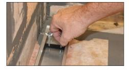
**(B)** Use the supplied height-adjustment aid to adjust the frame to the thickness of the tile covering.
