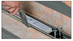
Use tile adhesive to fill beneath the frame on all sides and install the tile covering.
