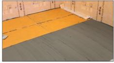
6 If DITRA uncoupling membrane, or DITRA-HEAT-E /-DUO underfloor heating is being used apply a bed of adhesive to the floor substrate and adhere DITRA uncoupling membrane, or DITRA-HEAT/-DUO.
