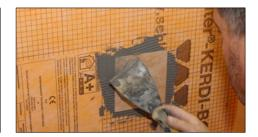
If Schlüter-KERDI-BOARD is used on the wall, use KERDI-COLL-L with a piece of KERDI-KEBA sealing band to waterproof the penetrations.
