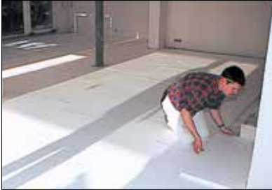
Installation of heat and/or sound insulation on a sufficiently load bearing and level substrate.
