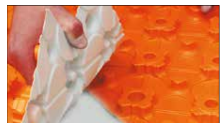
Laying out and fitting the studded screed panel Schlüter-BEKOTEC-EN 23 F
