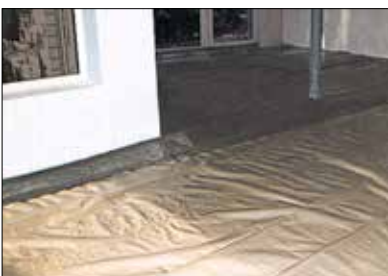
Installation of separating layer
