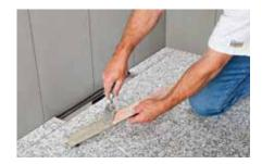
Schlüter-KERDI-LINE-D is a frameless channel cover to match Schlüter-KERDI-LINE channel bodies. The covering support features a fleece fabric for bonding with the tile adhesive and is universally suitable for all covering thicknesses.
