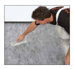
▶ 4. Use a float or roller to press Schlüter®-DITRA-SOUND fully into the adhesive.
