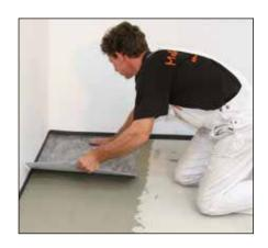
4 3. Lay Schlüter®-DITRA-SOUND mat into the wet adhesive, ensuring joints are tightly abutted.
