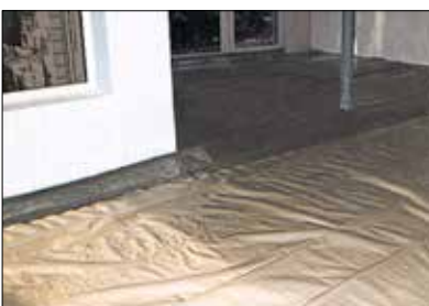
Installation of separating layer
