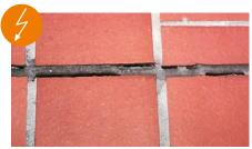
This type of damage is preventable with Schlüter®-DILEX movement profiles
