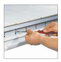
1. Schlüter®-BARIN gutter components are cut to size and connected to the Schlüter®-BARA profile with the screws provided. The slots allow the gutter to be sloped, if required.
