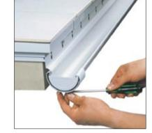
5. To connect a down pipe, a gutter section with on outlet of approximately 20 cm is attached with two clip on connectors, which are centred over the gutter joints.
