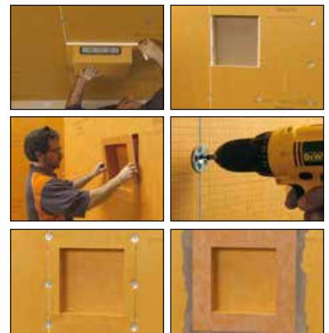
Installation in KERDI-BOARD
