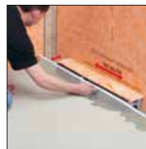
=> 4. Ajuster le support de caniveau
