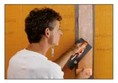
of individual construction requirements. Implement all connections with great care. Separate Schlüter-KERDI-BOARD above the existing movement joints and structural joints and cover the abutting joints with Schlüter-KERDI-FLEX. Schlüter-KERDI-FLEX is also recommended for flexible edges.
