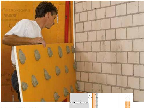
Schlüter-KERDI-BOARD can be fully adhered in wall areas or alternatively attached with dabs of adhesive. If necessary, the material may be secured with additional wall anchors. In the case of stud frames made of wood or metal, Schlüter-KERDI-BOARD is attached with screws from the matching hardware system.
