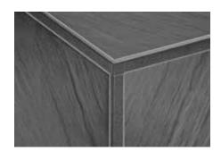
Corner connection with pre-fabricated corner piece
