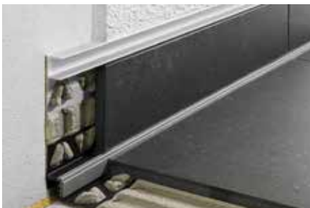
Installation in skirting
