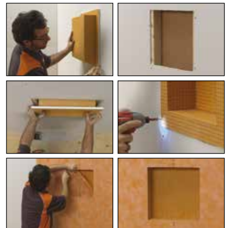
Installation in plasterboard
