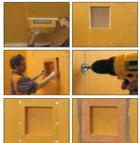
Installation in KERDI-BOARD
